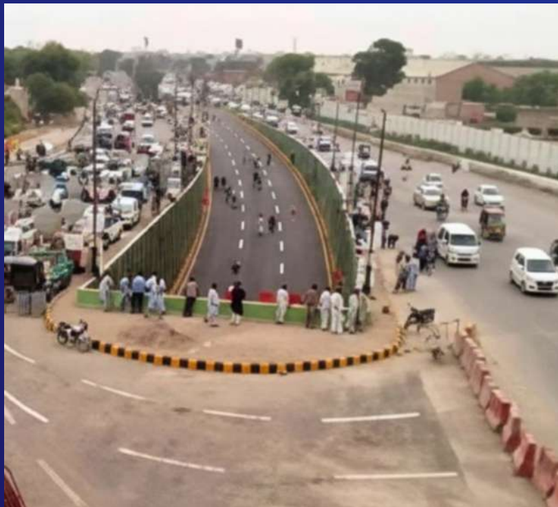
DRIGH ROAD UNDERPASS, KARACHI KMC JULY 2017
