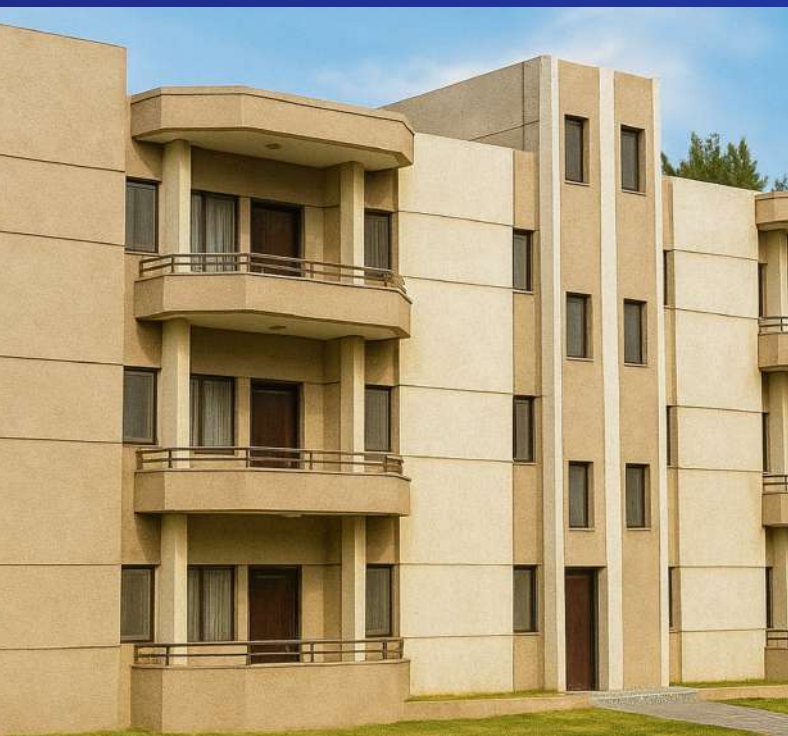
MULTI STOREY FLATS AT GOVERNOR HOUSE, SINDH GOVT OF SINDH OCTOBER 2017
