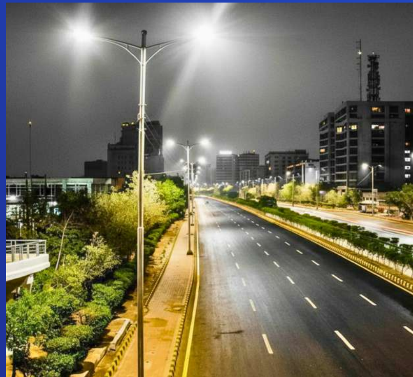
TARIQ ROAD REHABILITATION, KARACHI KMC JUNE 2017
